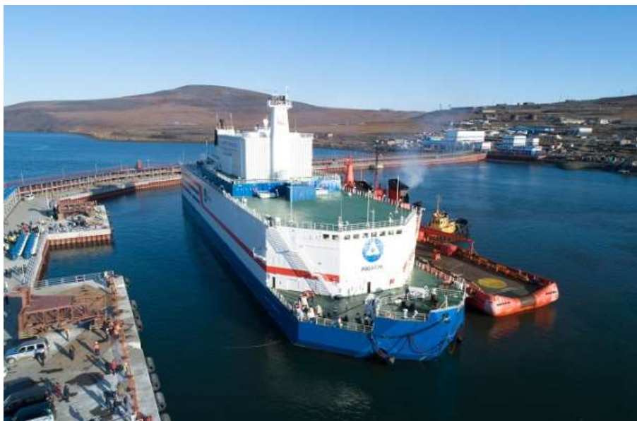
Fig. 3. The floating nuclear thermal power plant “Akademik Lomonosov”.
